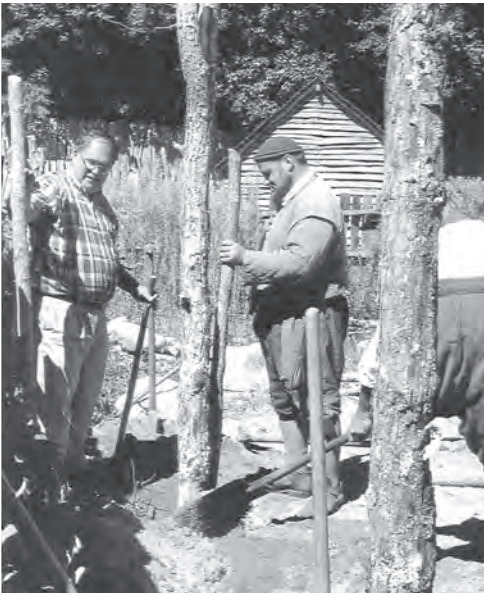
Jonathan Stubbs lends a hand in building the “new” Howland House at Plimoth Plantation.
