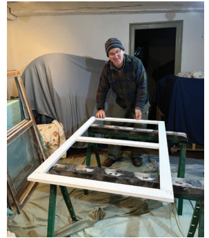
Executive Director Peter Arenstam repaired several windows.
