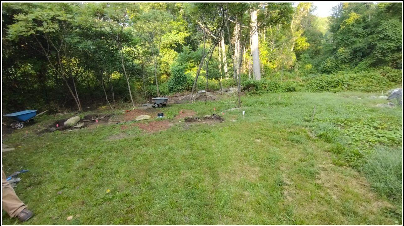
Figure 1. 2023 excavation area looking west.
